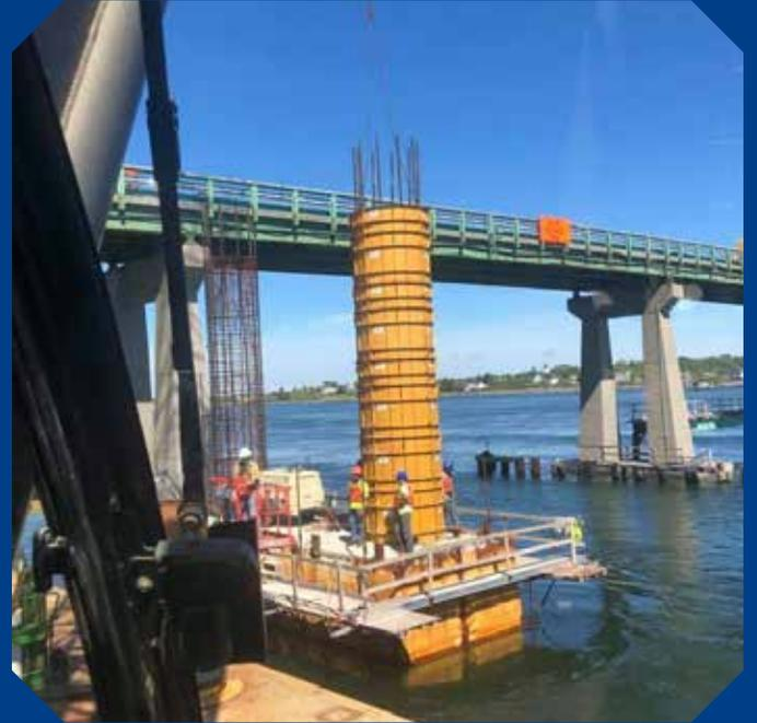
*Steel tube forms for new bridge cement pilings.*
