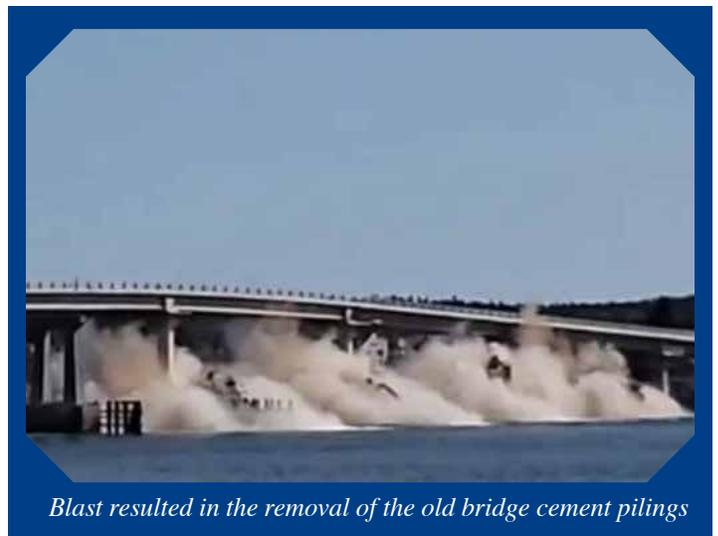
*Blast resulted in the removal of the old bridge cement pilings*
