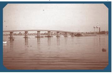
in the boxes. Once the concrete columns were built and the piers were finished the span could be completed. So, the bridge consists of steel pilings, concrete blocks, concrete columns, steel beams, decking, road surface, and railing materials, in addition to the approaches. The boxes are integral support components of the bridge span.
